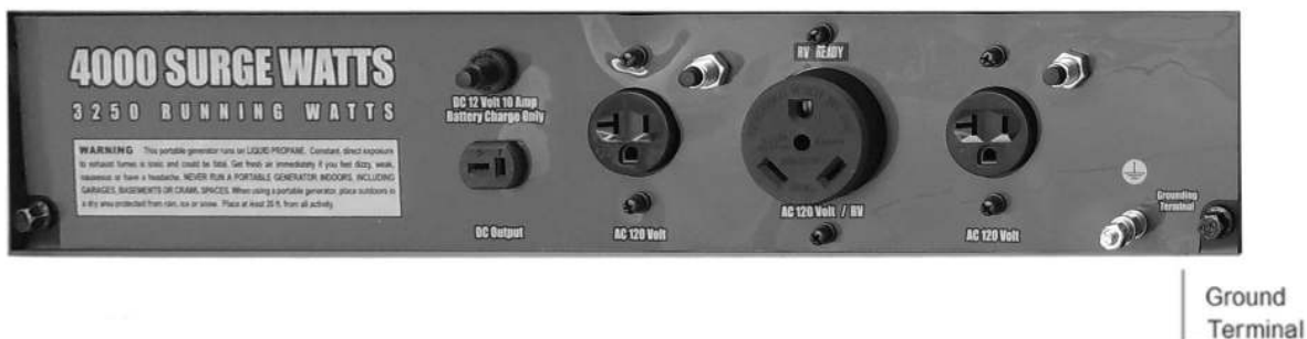
Figure 3 - Attaching the Grounding Wire to this Generator
